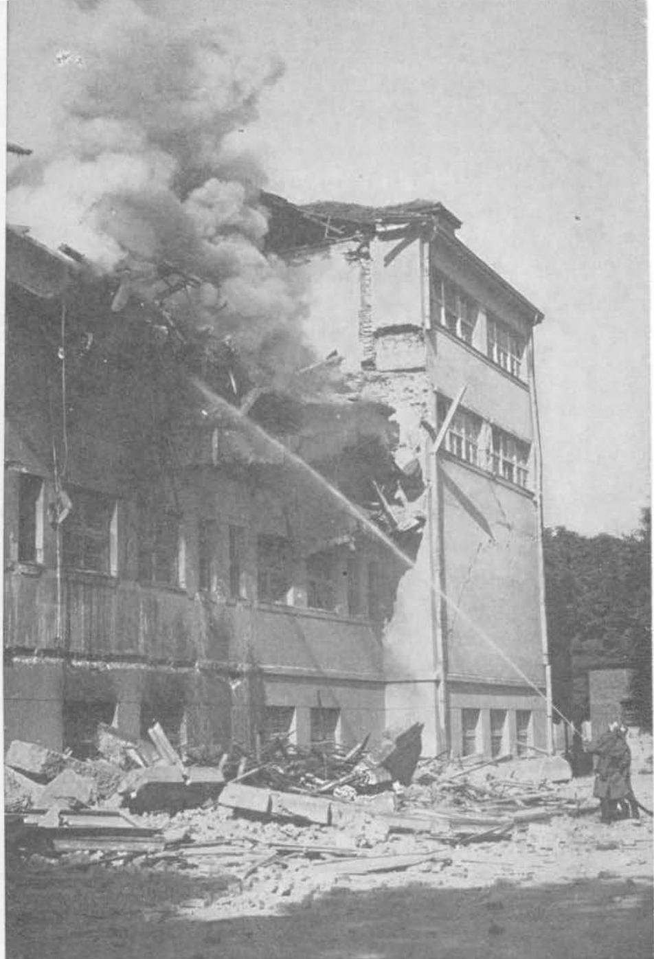
▲ THE SECONDARY POLYTECHNIC SCHOOL — EXTINGUISHING THE FIRE WHICH BROKE OUT IMMEDIATELY AFTER THE EARTHQUAKE.
