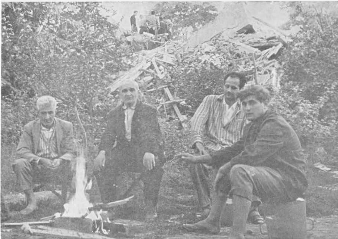
◀ THESE UNFORTUNATE PEOPLE BARELY ESCAPED ALIVE FROM THEIR HOUSE. THEY MADE A FIRE IN THE GARDEN IN FRONT OF THE RUINS AND AWAITED THE NEXT NIGHT WITH FEAR. IN SIX DAYS OVER 200 HUNDRED TREMORS WERE RECORDED IN SKOPLJE. SOME OF THEM WERE OVER FIVE DEGREES IN INTENSITY
