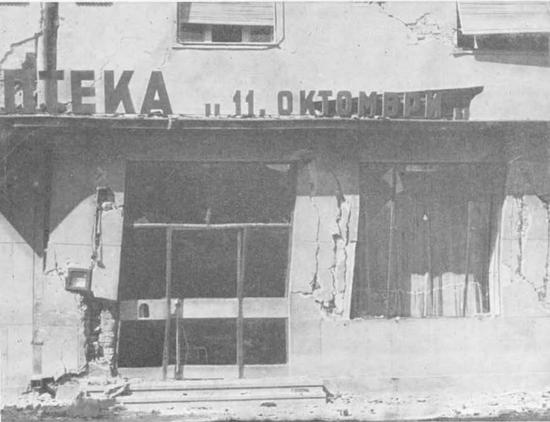
THE CENTRAL CHEMIST'S; NOT COMPLETELY DESTROYED, BUT BADLY DAMAGED AND BEYOND REPAIR.
