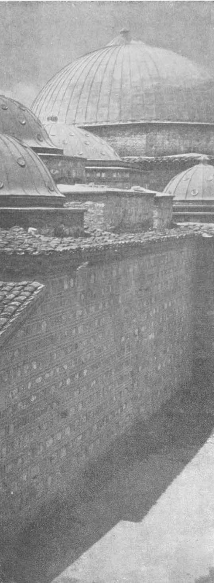
ONE OF THE MOST IMPRESSIVE MONUMENTS OF ISLAMIC ARCHITECTURE — DAUT PASHA'S BATH, PROBABLY BUILT IN 1489. — IS SITUATED BY THE STONE BRIDGE OVER THE VARDAR. THE BUILDING, WHICH CONTAINED AN ART GALLERY, WAS CONSIDERABLY DAMAGED.
