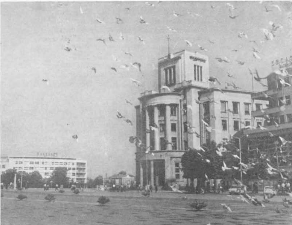
THE NATIONAL BANK ON MARSHAL TITO SQUARE BEFORE THE EARTHQUAKE. IT WAS BADLY DAMAGED. ◀
