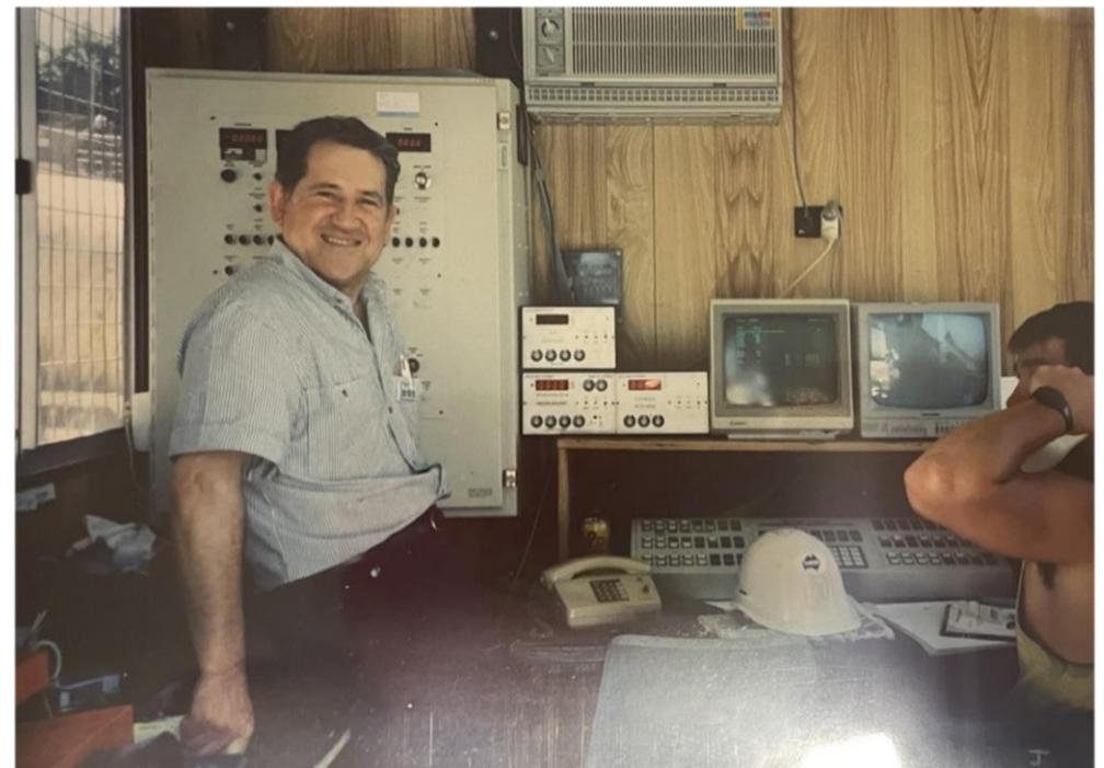
A proud Tony in the Batch room of the onsite concrete mixing plant with a Manu Electronics **ME188** controllers interfaced with PLC/Computer system.
